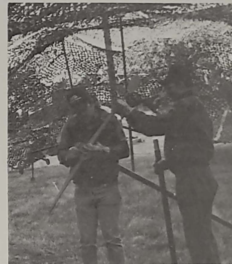
While others on the DSMT finish staking down and sandbagging the camouflage netting, TSgt. Dennis Smith and TSgt. Charles Pospisil adjust the fan braces that elevate the netting to keep it clear of personnel and equipment. (USAFR photo)
